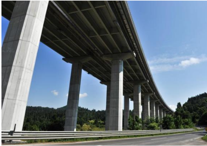
Ravbarkomanda highway bridge in Slovenia
